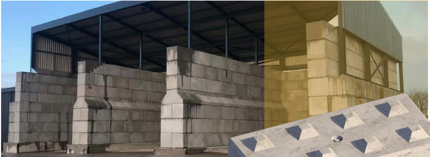
When designed and installed correctly they can form very large walls that take large loads. The use of double thickness walls at the base allows the walls to take the product loading and impact loading of the operating machinery with ease. With the division walls, a "footblock" is used which creates a very neat detail and is also self-cleaning of material.
